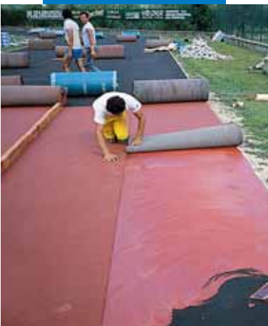
Installing rubber flooring with Adesilex G19
