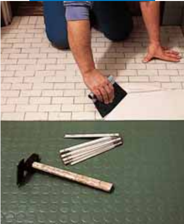
Spreading Adesilex G19 with a notched trowel
