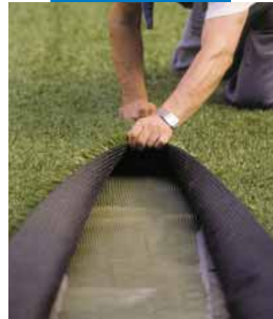
Installation of synthetic grass flooring with Adesilex G19 - S.Siro Stadium - Milan - Italy
